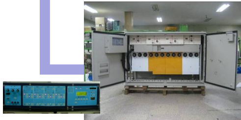
Pad mounted Switchgear
