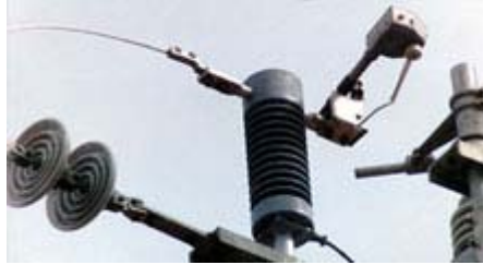
Overhead Current and Voltage Monitoring Insulators (CVMI)
