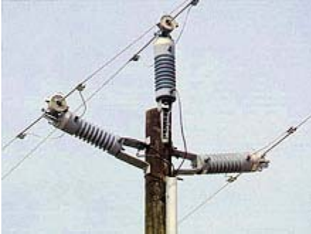
Overhead Current and Voltage Monitoring Insulators (CVMI)
