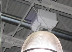
When the lights are brought back on, there is an extended period where they heat up to turn on and reach full brightness. During this time, errors were registered adding up over the time period:
