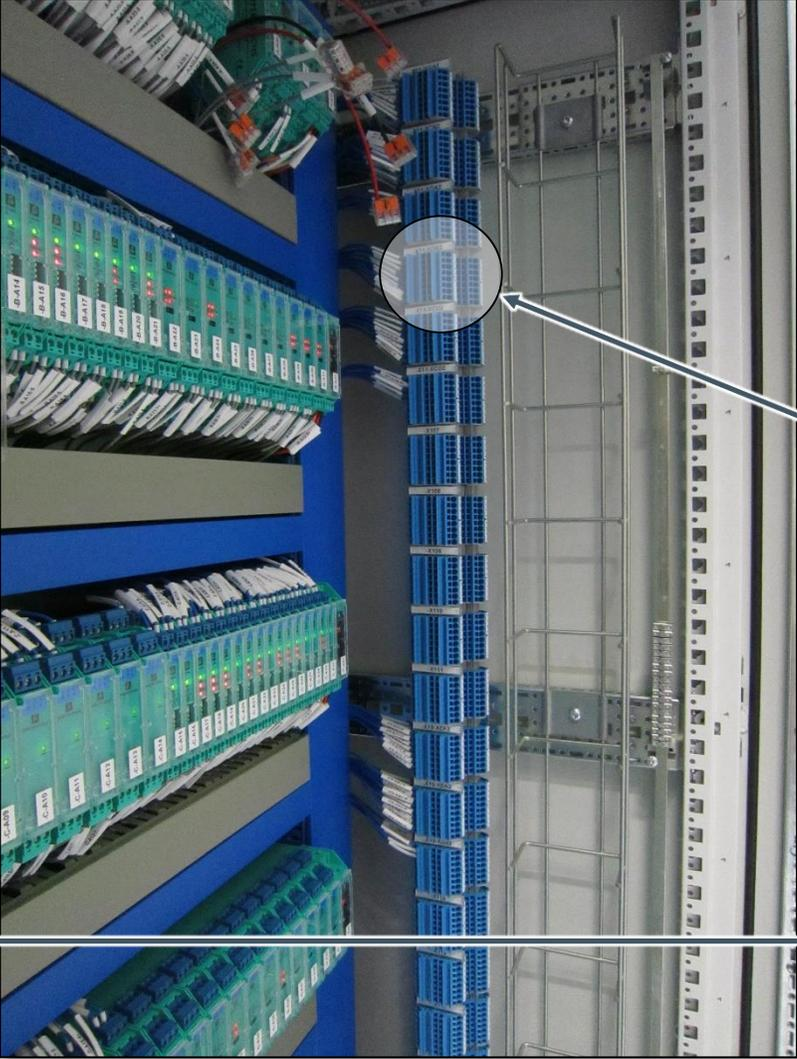
Inline connectors (junction terminals) just a short distance after the device ports to allow pre-manufacturing of the cabinet and easy cable installation at the construction site.
