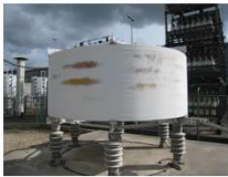
Surface condition which requires re-painting
