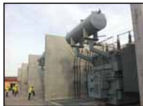
A row of transformers which will be enclosed inside the downtown substation building.
