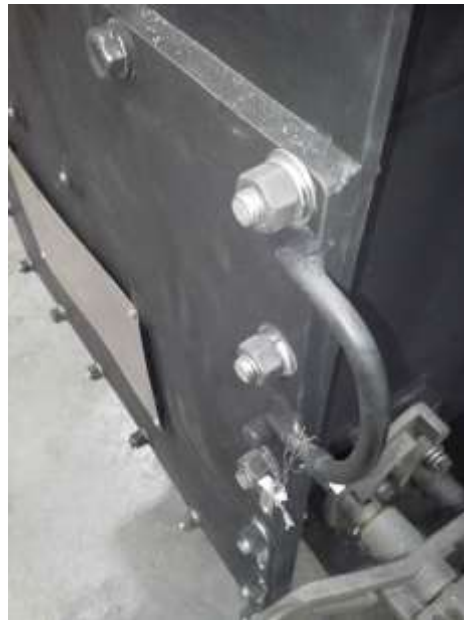
Figure 13: 300-Series Stainless Hardware on Steel Enclosure
