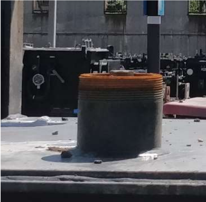
Figure 6: Brass Pipe Cap (not shown) on Steel Pipe
