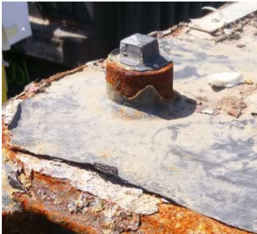
Figure 11: Brass Pipe Plug on Steel Threads
